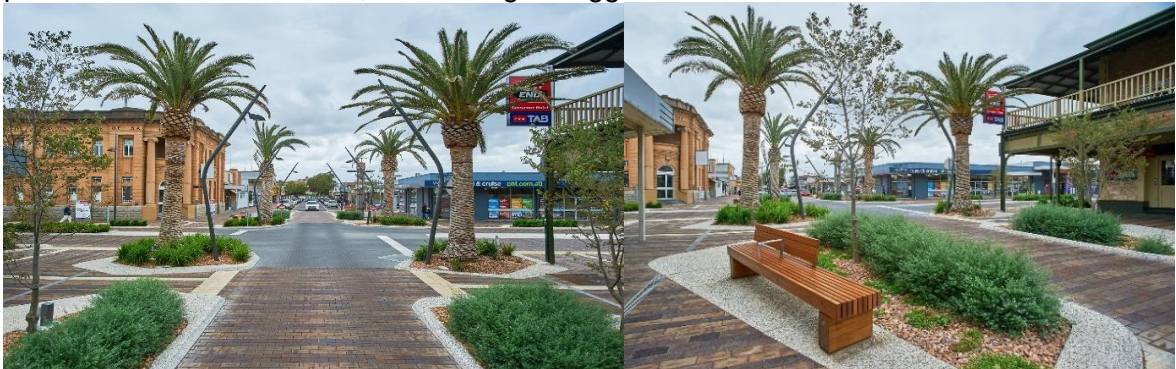
Images of the completed Stage 1 of the Mainstreet Upgrade.
